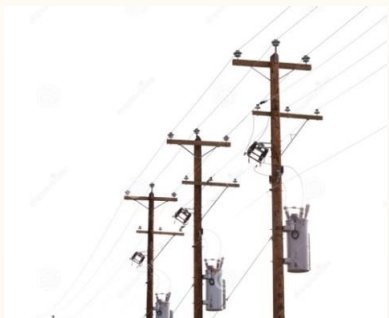
Distribution Wood Poles
