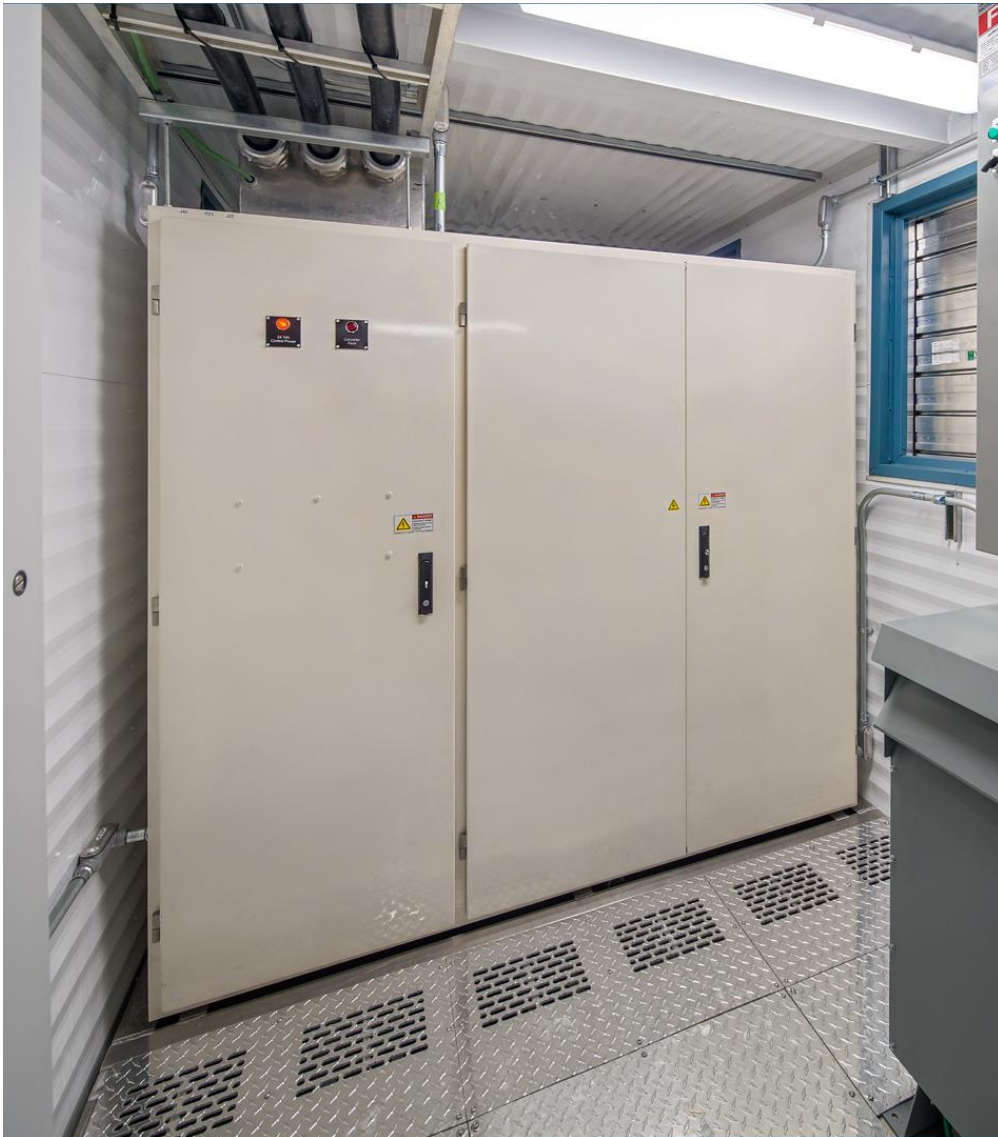
Interior Electronics Room- Arctic Containerized Package for NTPC- Converter, and exterior mount HMI
